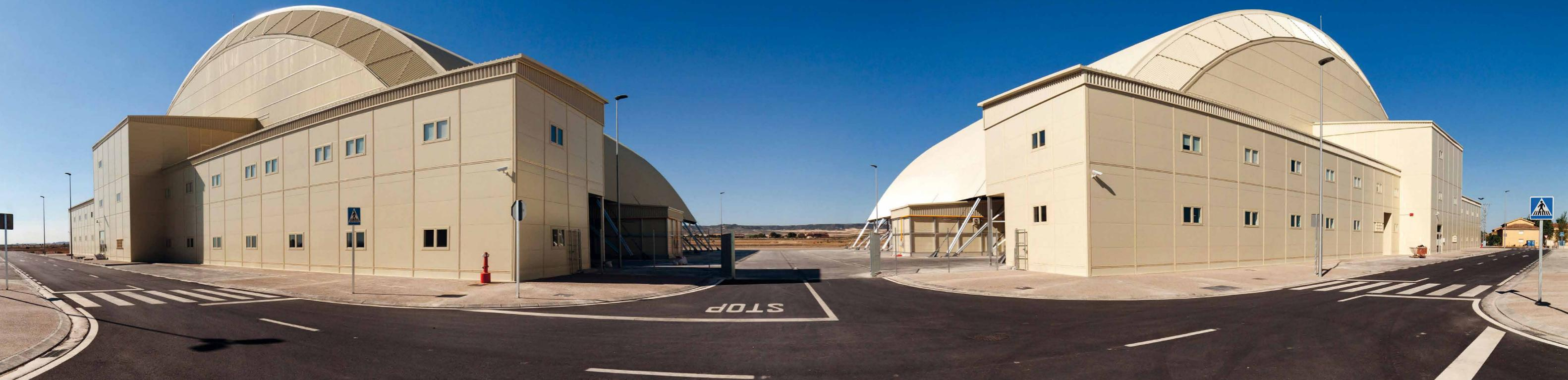
**The structures are composed of structural aluminium profiles with mechanical joints.**
